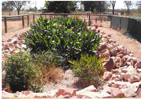
Figure 5. One of the five Wastewater Gardens systems at Pandanas Park Aboriginal community, Derby, West Australia. This one receives the effluent from three individual house septic tanks. The system is a “sunken garden” so that gravity-flow is sufficient to bring wastewater to the inlet pipe. Shown here after its first year growth.
